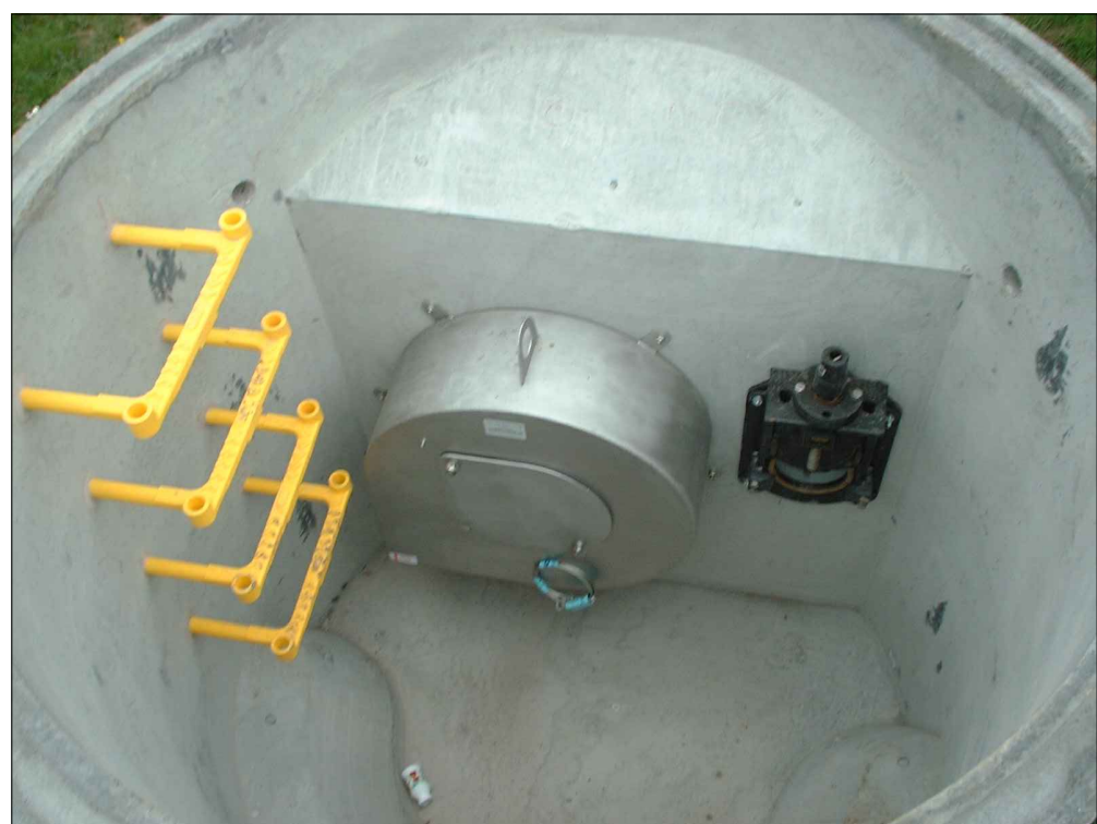
VIEW OF HYDRO-BRAKE & PENSTOCK VALVE AS SUPPLIED BY CPM SCALE 1:20
