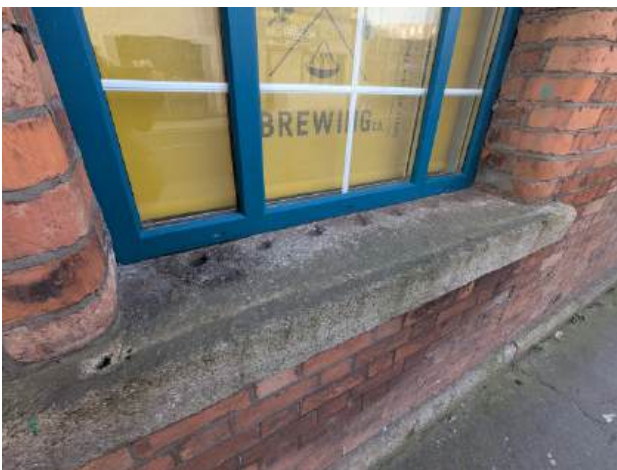
Window guard rail holes in sill
