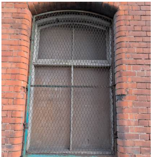
Historic metal-framed first floor windows c. 1920s-1930s, however some of these in the east probably date to pre-1916
