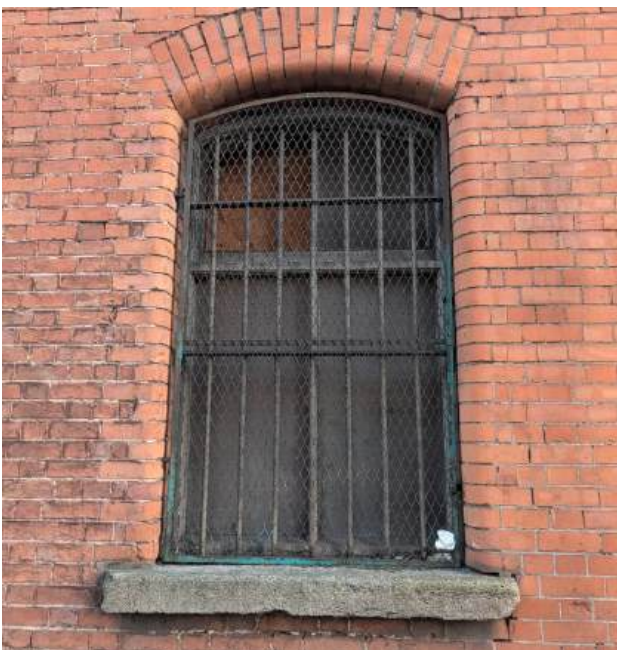
Historic wooden frames in eastern ground floor windows c. 1886-1900s
