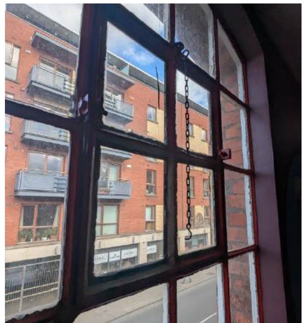
Historic metal-framed first floor windows c. 1920s-1930s, however some of these in the east probably date to pre-1916
