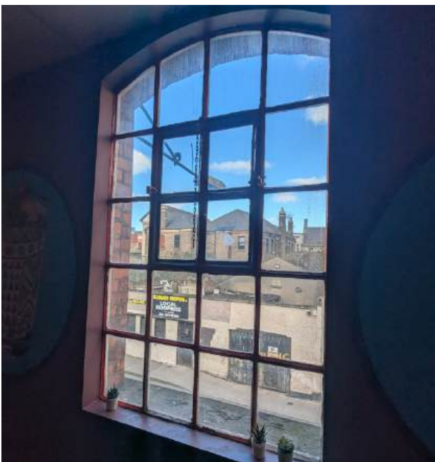
Historic metal-framed first floor windows c. 1920s-1930s, however some of these in the east probably date to pre-1916
