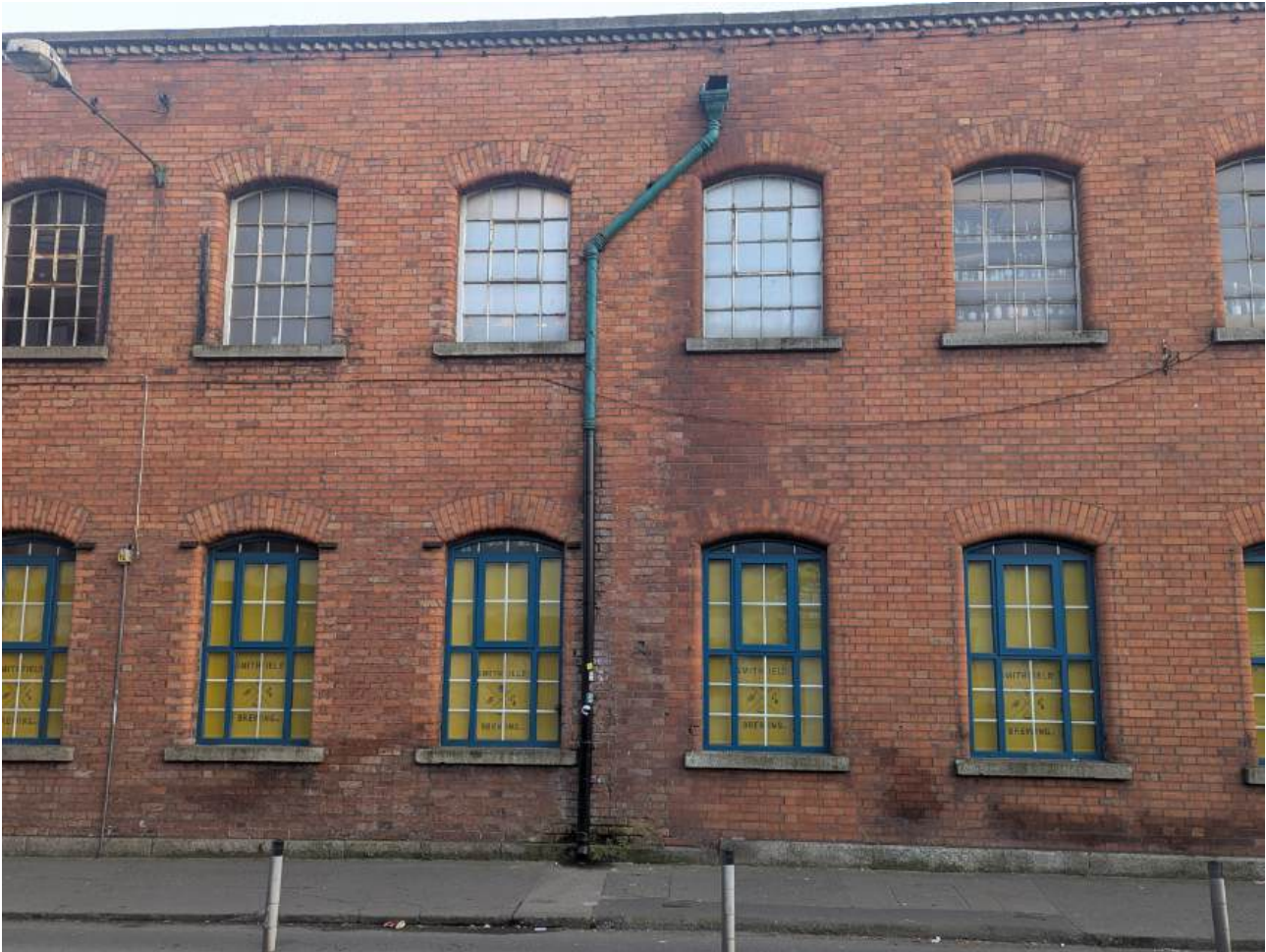
Change between 1886-1900 phase of building (left half) and 1920s phase (right half), note change in brick
