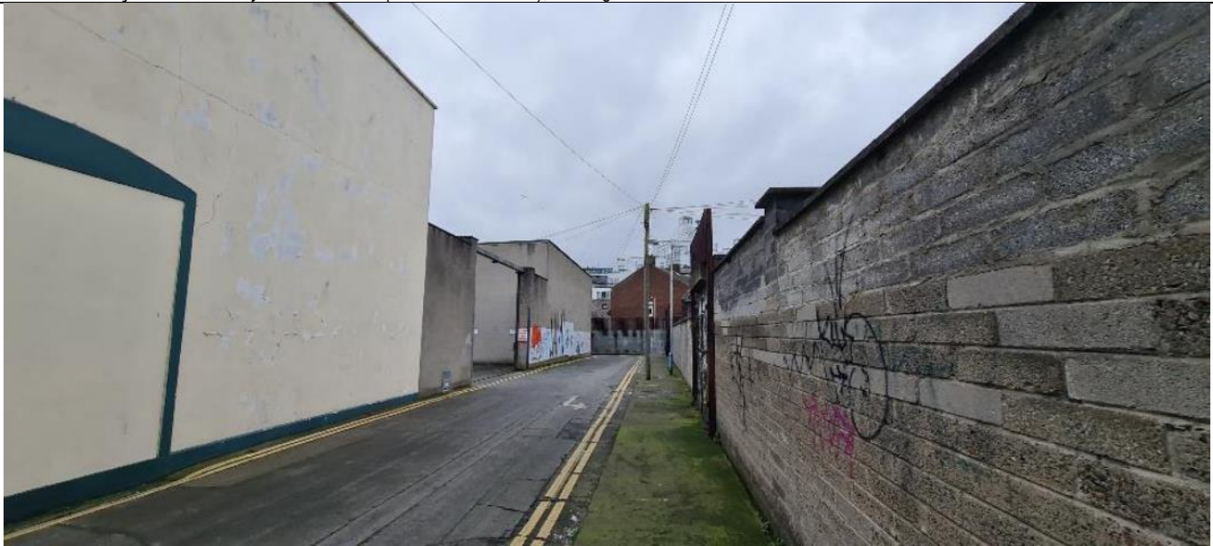
Fig. A13 West frontage of site onto Brown Street
