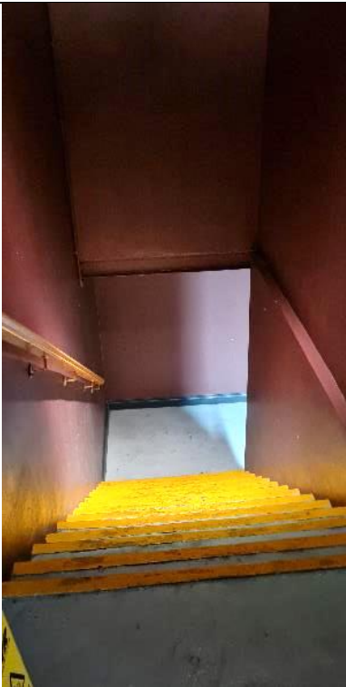
Fig. A55 First floor, staircase
