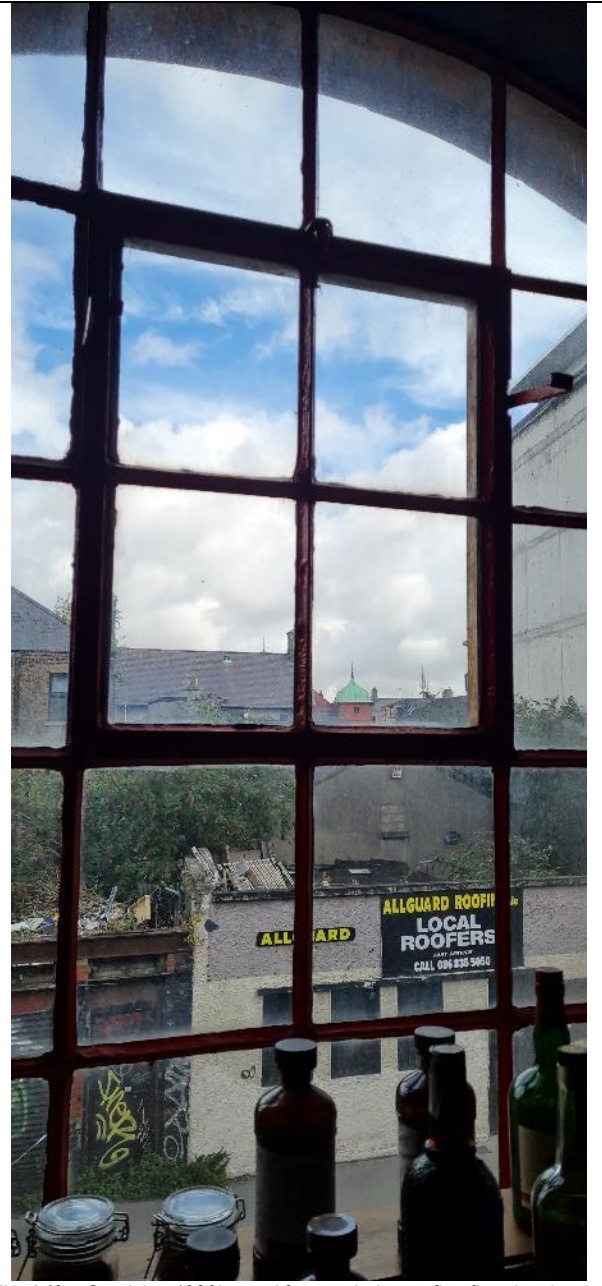
Fig. A49 Surviving 1920's steel frame window at first floor level
