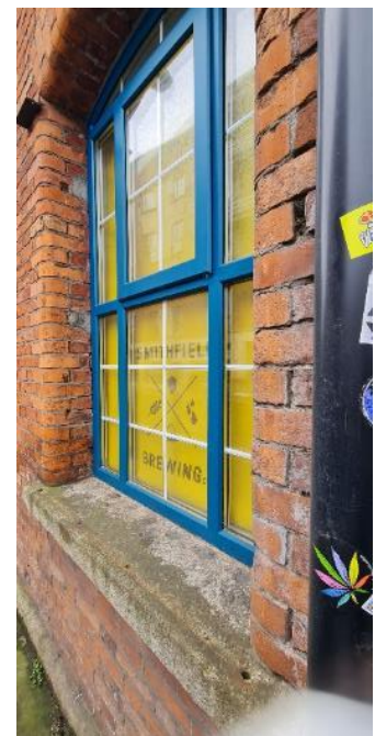
Fig. 15 Ground floor window opening on central section of facade
