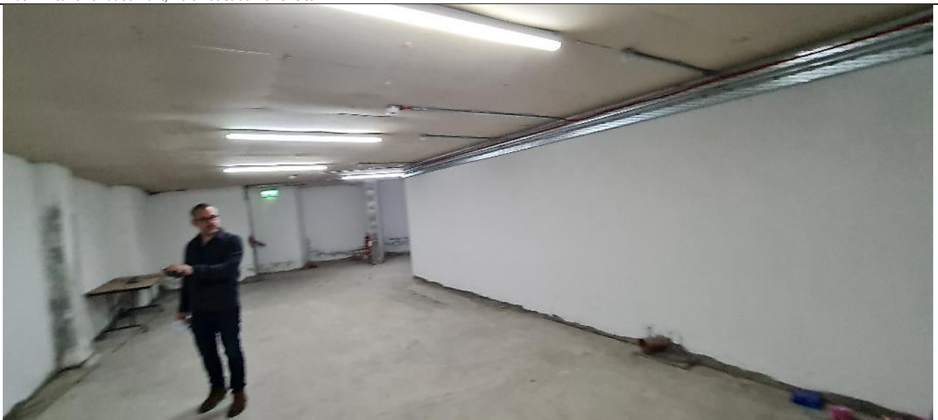
Fig. A64 Interior of basement, north-east corner of site
