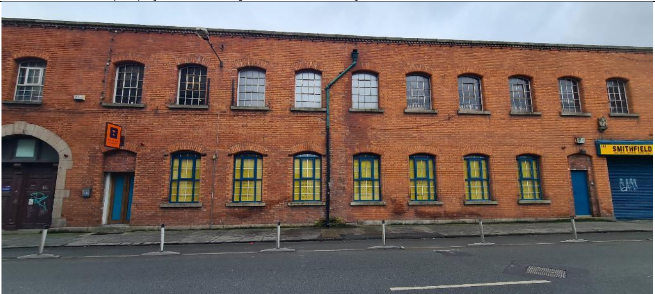
Fig. A2: Central section of front (north) façade onto North King Street. The façade to the left of the downpipe dates from c.1885. The façade to the right forms part of the 1920's extension by Jones & Kelly.
