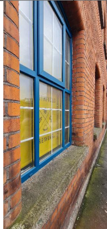
Fig. A10: Detail of ground floor opening with replacement window on central part of façade (c.1923)
