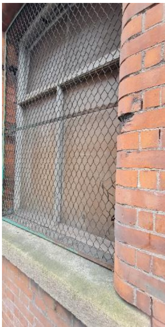
Fig. 13 Ground floor window on eastern part of facade
