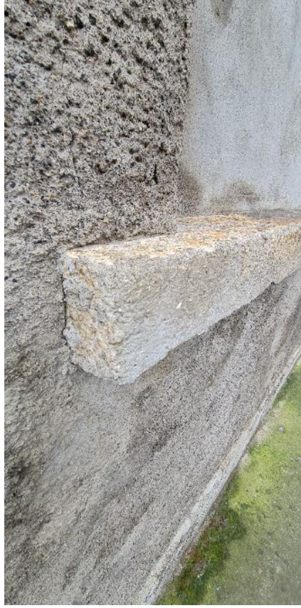
Fig. A22: Granite sill on east façade (Bow Street)
