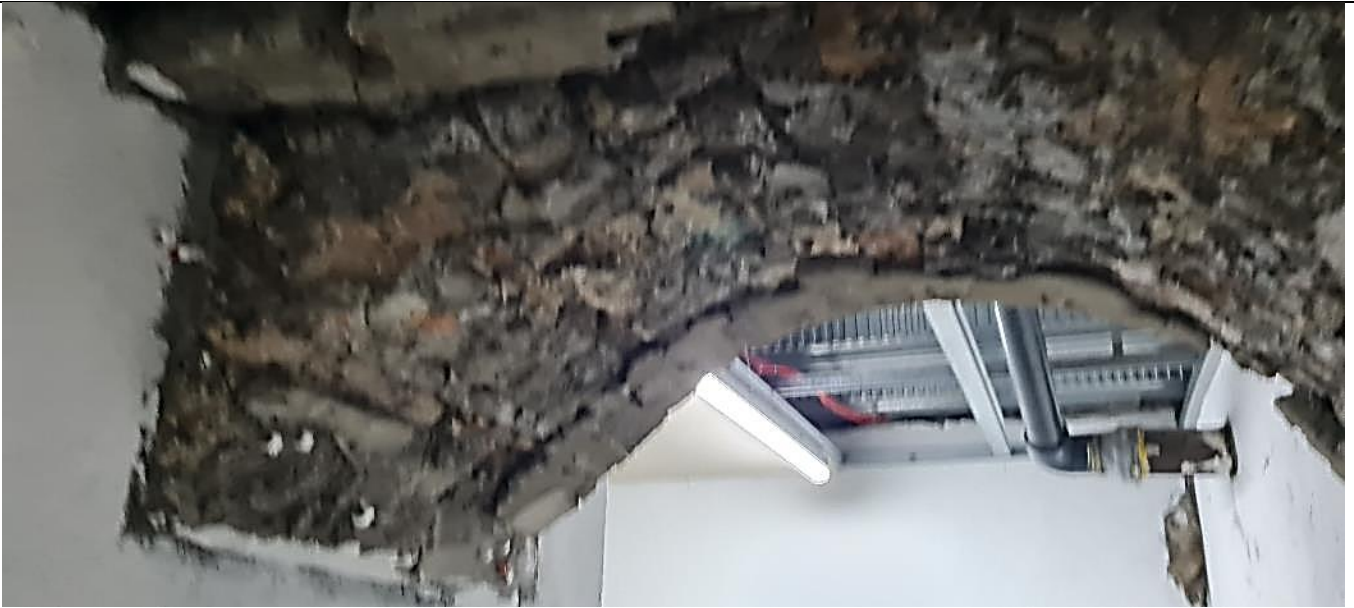
Fig. A65 Brick arch, interior of basement, north-east corner of site
