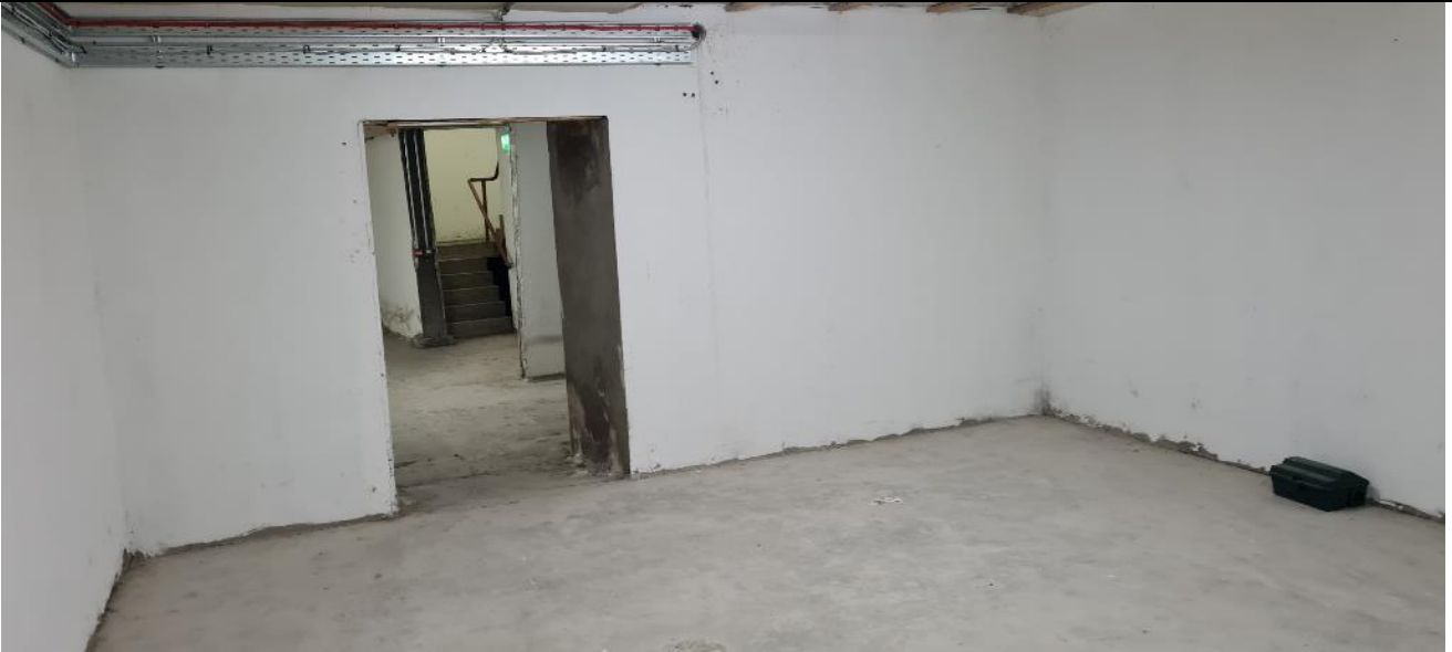
Fig. A62 Interior of basement, north-east corner of site
