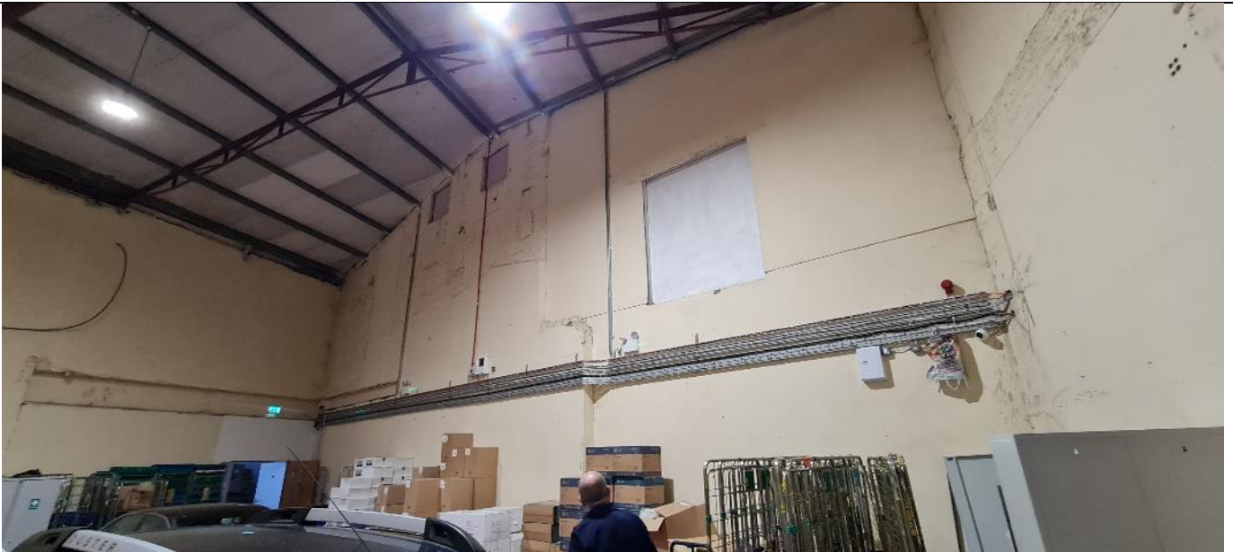
Fig. A38: Interior of warehouse off Bow Street, at south-east corner of site
