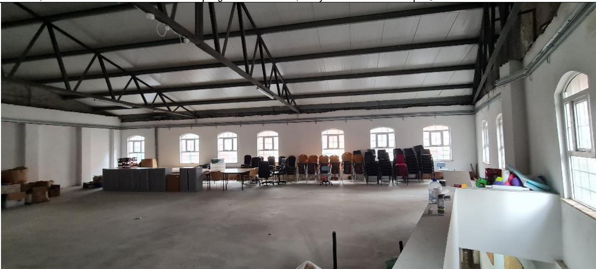
Fig. A58 First floor, north-east corner of 139-149 North King Street
