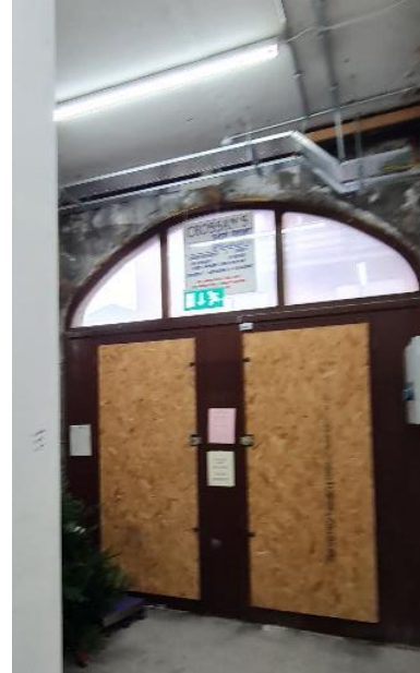
Fig. A44 Modern doors within former carriage arch on north external wall
