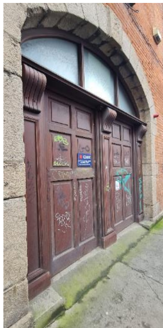
Fig. 14 Former carriage arch with modern panelled timber door
