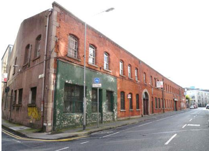
Fig 11 Photograph of front façade onto North King Street (NIAH Survey)
