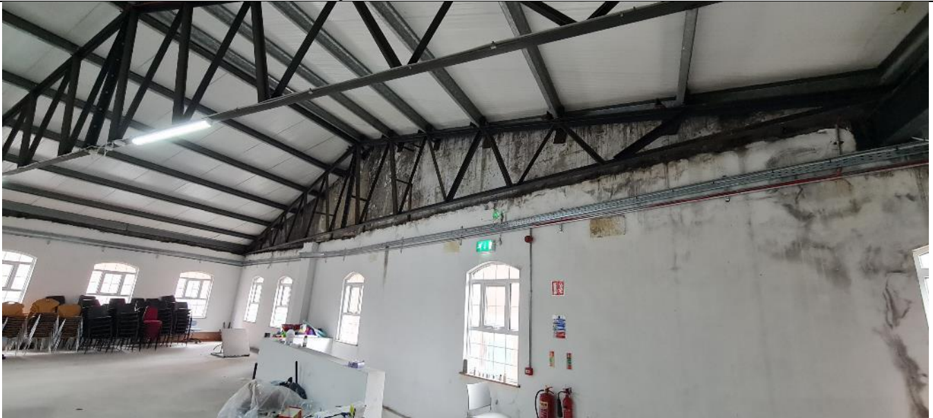
Fig. A60 First floor, north-east corner of 139-149 North King Street
