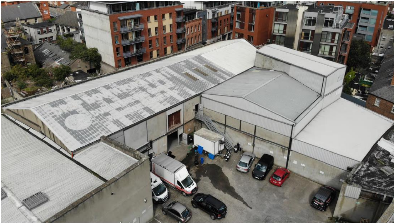
Fig. 21 Drone photograph (April 2023) looking north-east showing modern roofs and warehouses to the rear of the retained north and east facades.
