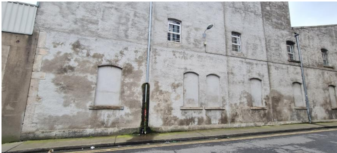
Fig. 17 Southern portion of the east façade onto Bow Street, with blind openings at street level and windows to the first floor opening. The granite plinth and granite quoin (to the south corner) suggest that the entire façade (ground floor level at least) dates from the construction of the late-nineteenth century soap factory.
