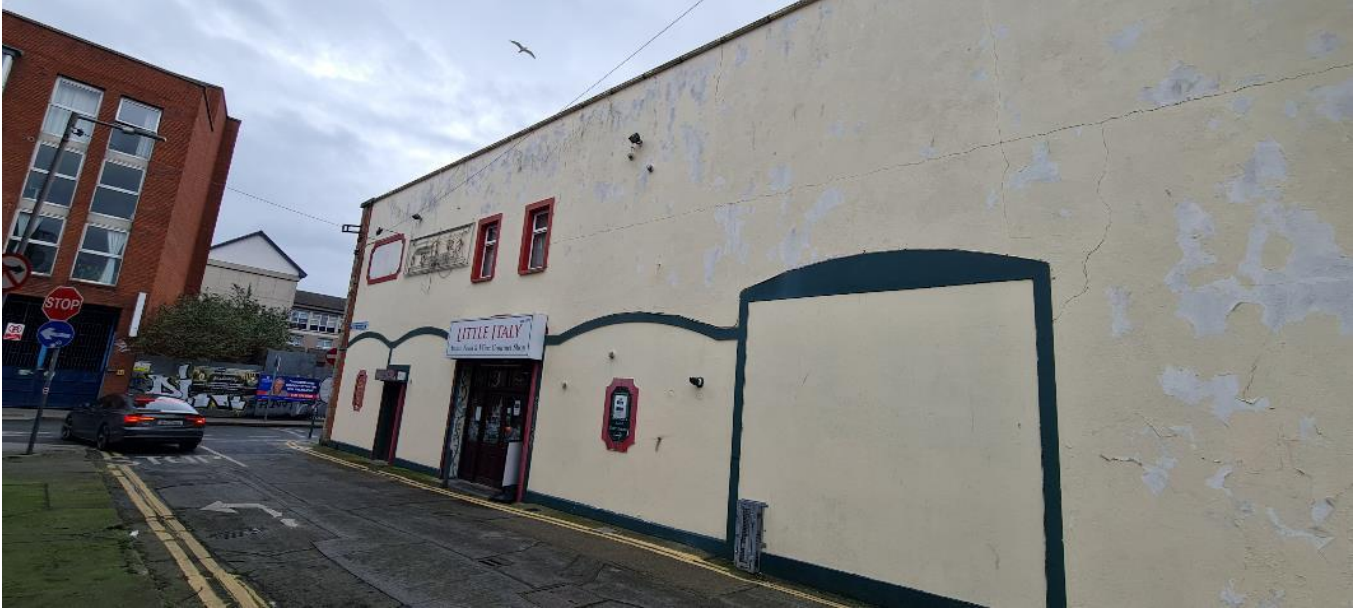
Fig. A12 West façade of 'Little Italy' wholesale unit (constructed c.1994), fronting onto Brown Street
