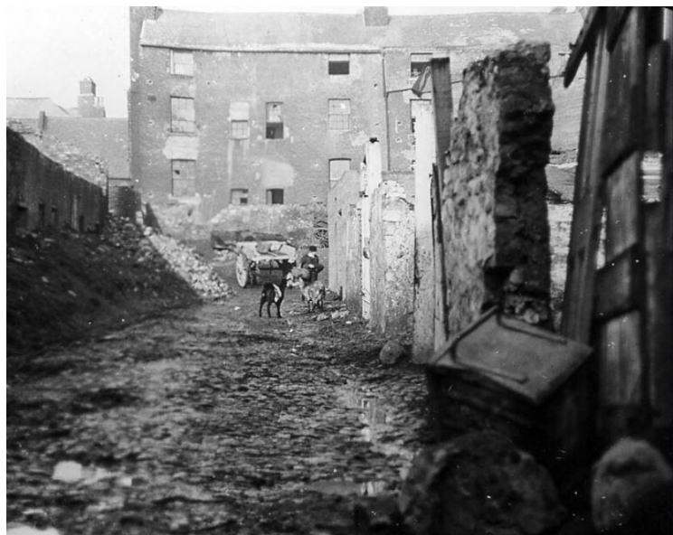
Fig. 4 Historic photograph of Cavanagh's Court showing the four-storey rear (south) facades of 141 and 142 North King Street prior to their demolition
