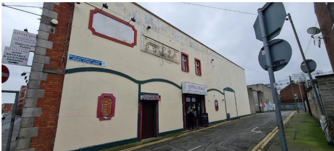
Fig. 18 West façade onto Brown Street
