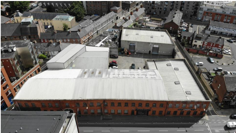
Fig. 9 Recent aerial photograph looking south towards 149-139 North King Street. This photograph shows the modern metal deck roofs to the rear of the retained brick façade (reproduced from Architectural Design Report by MOLA)
