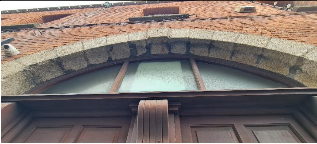
Fig. A8 Detail of granite reveal to former carriage arch on front (north) façade. The paneled timber doors are a late-twentieth century infill
