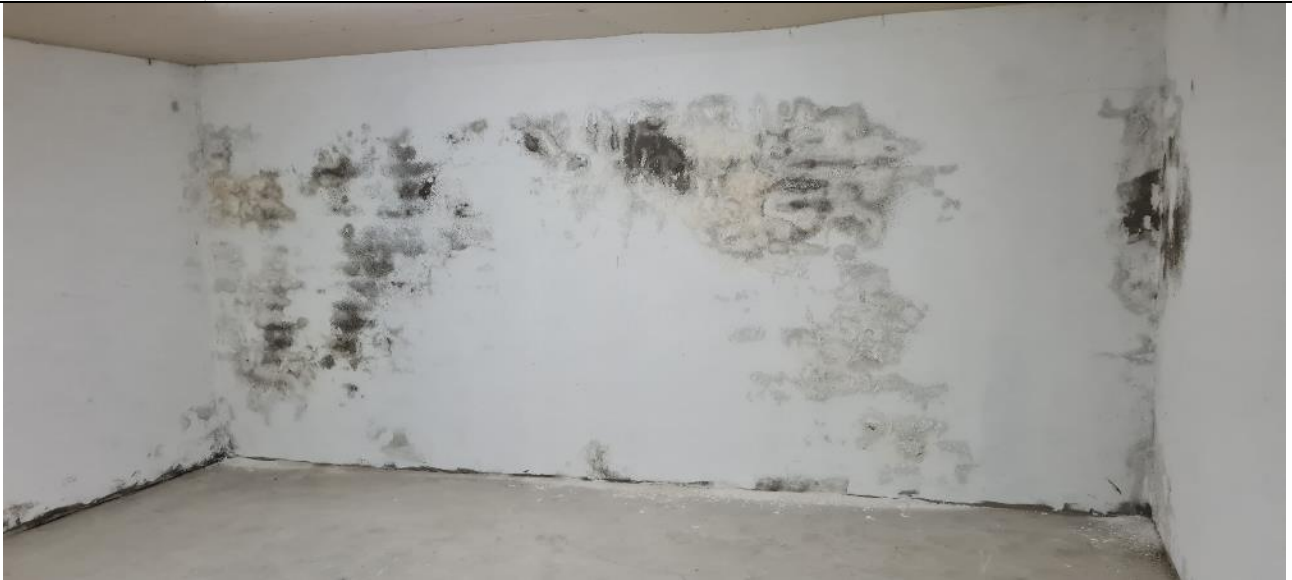
Fig. A63 Interior of basement, north-east corner of site
