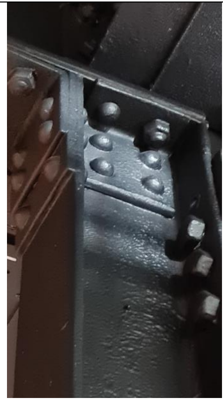
Fig. A36: Detail of steel column in microbrewery
