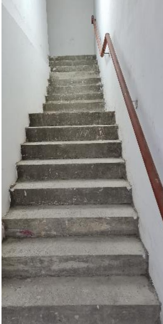
Fig. A43 Staircase to first floor at north-east corner of site
