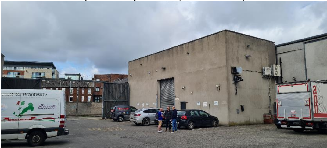
Fig. A25: Goods yard to rear of 139-149 North King Street – view looking west towards Brown Street
