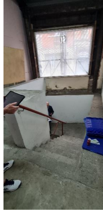
Fig. A42 Staircase to basement at north-east corner of site
