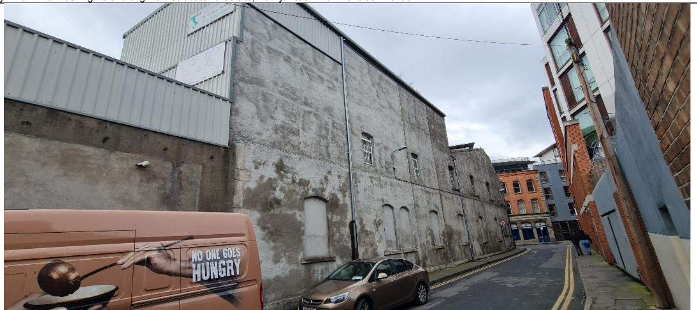
Fig. A17 East frontage onto Bow Street. Sections of this warehouse façade date from the construction of the former soap factory in c.1885
