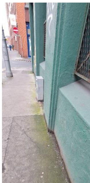
Fig 12 Cement-rendered shopfront at eastern end of façade to North King Street
